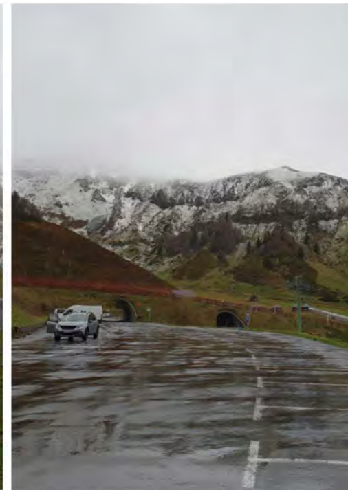
SITE N° 4 : PARKING PRINCIPAL
